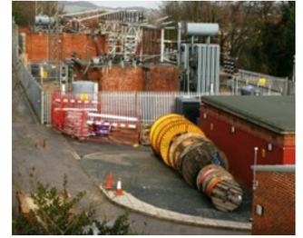
'The 34-tonne transformer, crane and other equipment was delivered across the main Hastings to Charing Cross railway line' (from Upper Grosvenor Road) 'on consecutive nights, while trains were not operating. A second transformer will be delivered to the substation in February, then further work will take place inside the site to test, connect and make the equipment live.'
