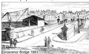
The bridge was opened on March 7th 1883 by Mrs Stone-Wigg (wife of the Chairman of the Local Board) and the Kent & Sussex Courier included a special section. The bridge was constructed with three ironwork spans supported on red brick piers, with three 12ft arches under each of the approaches. These arches were intended to be let out as storerooms but three became the town mortuary and others were used by the Local Board for storage.
